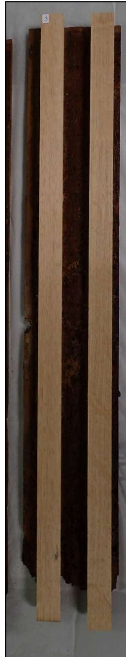
Overview of back showing specially designed ribbed tulip wood battens designed by Hugh Harrison FSA and made by conservation joiner Stuart Anderson.
