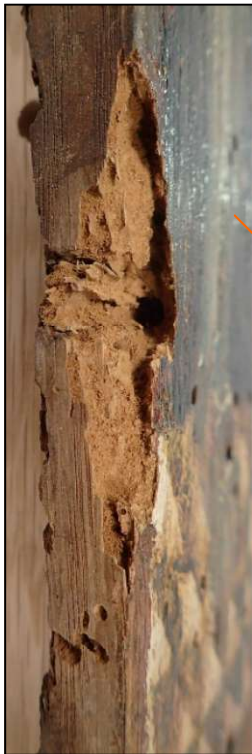
Above and below, details of the fragile edges. In places the surface was held together solely by the paint layers.
