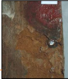
Detail showing powdery wood and beetle frass.
